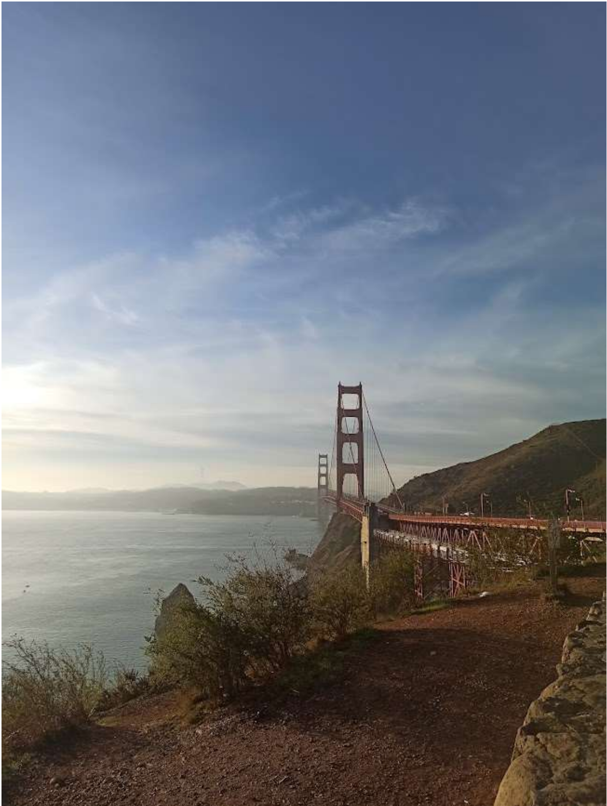
Golden Gate Bridge – San Francisco
